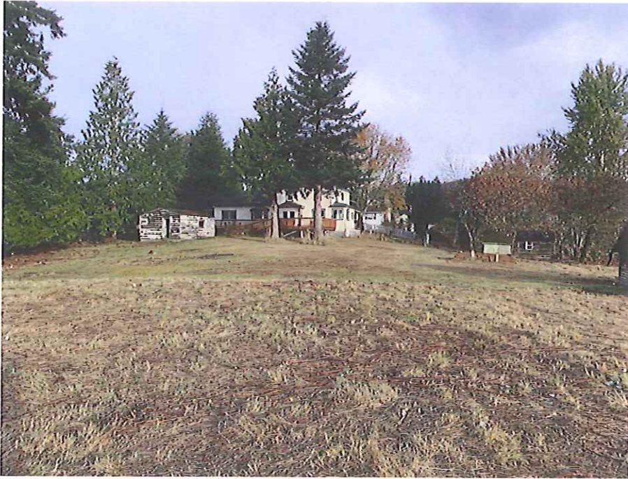
Photo 5. View north from the south property boundary over the house (11/1/22).
